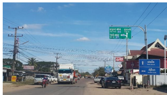
Figure 6. Road Infrastructure in Thanaleng
